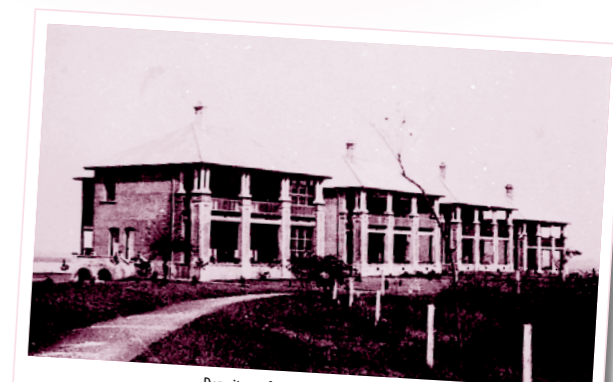
Dormitory of LTS in Shekou, Hubei Province.
